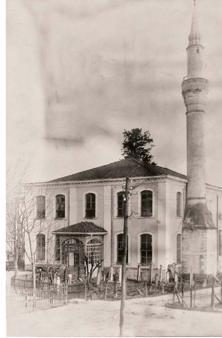
Adapazarı'nda Sultan Orhan Camii Şerifi / 1901 Sultan Orhan Mosque in Adapazarı
